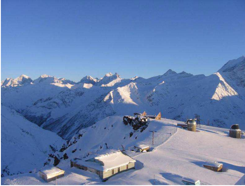
Fig. 5. The old hotel and the small telescopes - a view from the 2-m telescope dome
