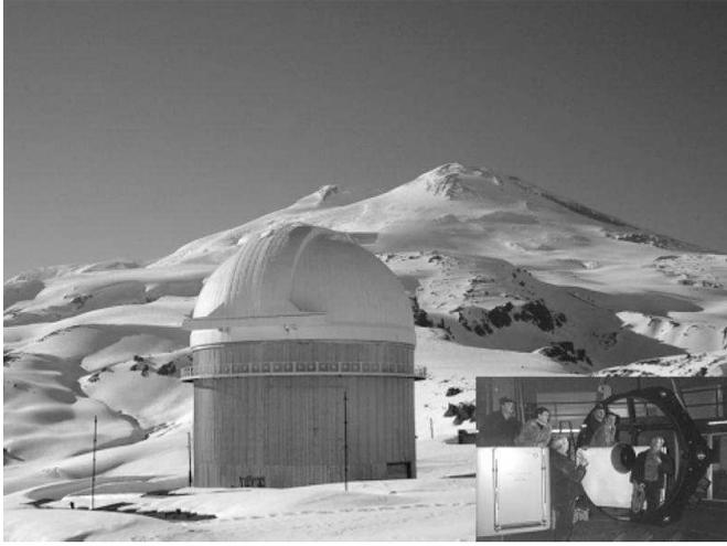
**Fig. 4.** The dome with a 20 m diameter and the 2-m mirror of the RCC telescope
